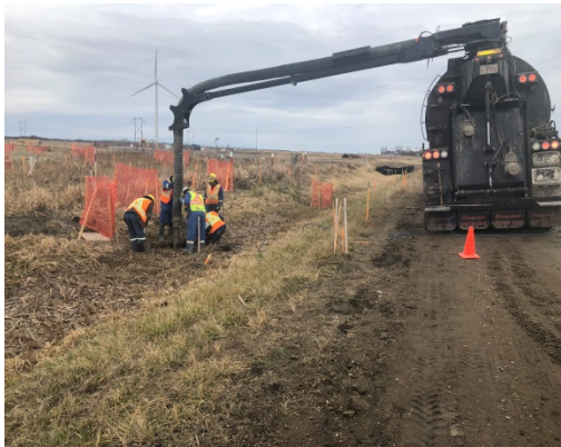
SF 47, photo facing north, crews hydrovacating to locate the drillers drill bit.
