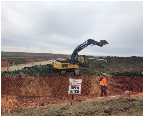
SF 43A, photo facing east, excavator digging hole for where pipe will go under the road.
