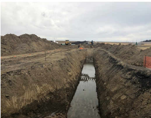
SF 42, photo facing west, excavator moving dirt out of the trench onto the ROW, one dozer then moving that dirt to the side of the ROW.
