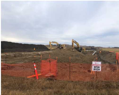
SF 33, photo facing west, excavators backfilling pipe.
