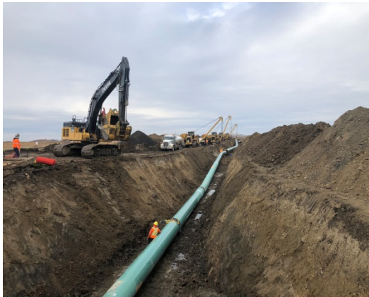
SF 35, photo facing west, crews tying in the pipe.
