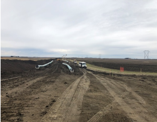
SF 44, photo facing west, side booms moving pipe closer to the trench.
